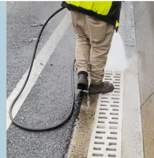
7. Clear the grate frame of debris and bolt the grate to the access channel.
