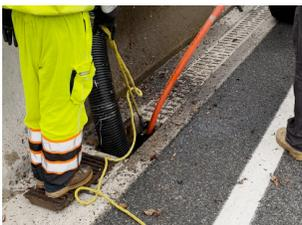
4. Insert vacuum hose and 360° pressure jetting hose from vacuum truck into the access channel opening.
