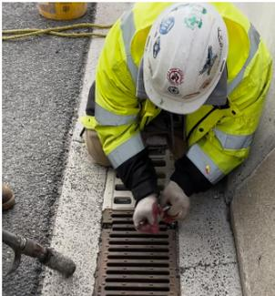
3. Remove the 4 bolts in the HD200 Access Channel with a 15 mm socket.
