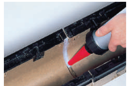
Sealant applied with caulk gun
