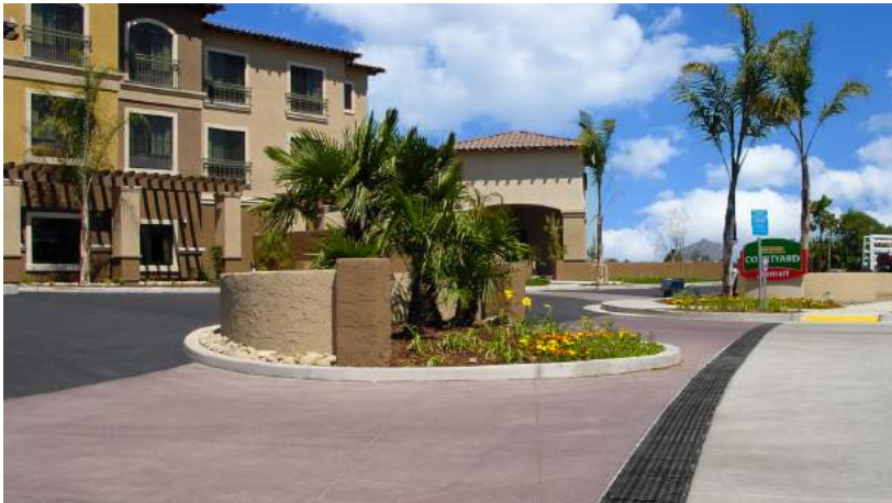
1. Linear Drains - Typical example of a correct, well-installed linear drain.
