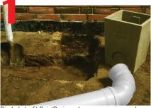
Dig hole to fit PointDrain and necessary pipe-work.
