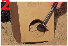
Drill out/cutout holes for pipe connection.
