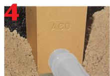
Connect drainage pipe, check for leaks before backfilling.
