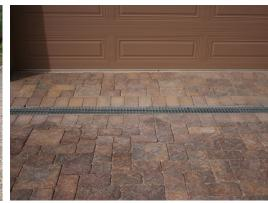
In-line polymer concrete catch basin
