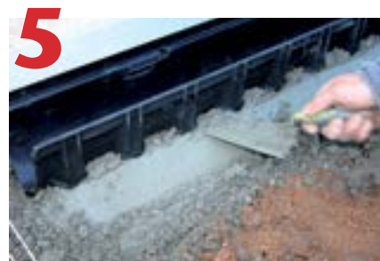
Lay 4" deep concrete bed. Lay channels working away from outlet. Concrete surround should extend up channel sides into recesses to hold channel in place.
