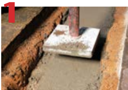
Excavate area to accommodate trench drain and 4" concrete surround, compact base.
