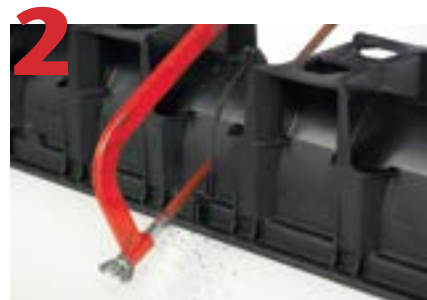
Cut channels to fit required length (if necessary).
