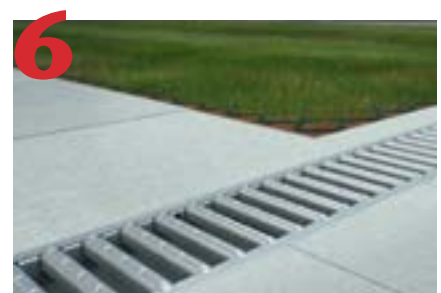
Finish pavement/pavers must be 1/8" higher than the grate.
