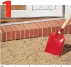
Excavate area large enough to fit DrainMat base, add 2" sand and compact well.
