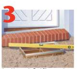
Level base unit. Backfill surround with concrete and finish surface as desired (tile, paver, etc.).
