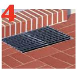
Ensure finished surface is 1/8" higher than the DrainMat to assist water drainage. Fit mat into finished installation.
