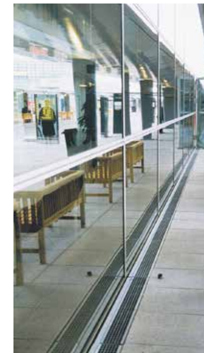
Membrane collects liquids that seep through surface materials.
