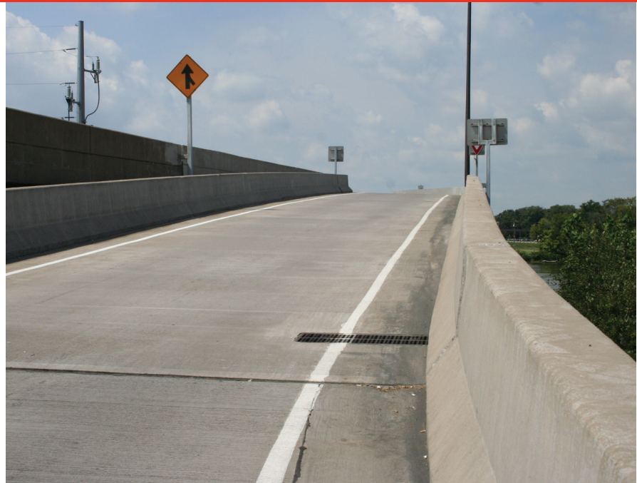
8" internal width fiberglass scupper for bridge deck drainage.
