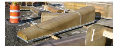
When compared to a traditional cast-inplace trench drain with special epoxy coatings an Aquaduct FRP trench drain can offer significant cost and time savings.
