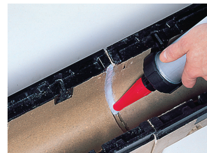
Sealant applied with caulk gun
