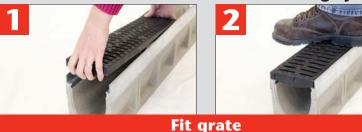
Position grate onto channel, align anti-shunt detail with recess in rail.
